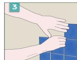
3 Press tile into properly placed setting material.
